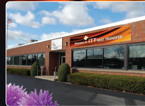
ITT Standard is headquartered in one of the largest and best-supported heat exchanger centers in the world.
